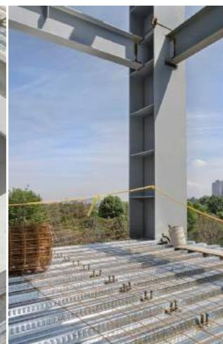
**DẦM THÉP LIÊN HỢP VỚI SÀN BÊ TÔNG, TẤM SÀN VÀ ĐINH NEO**
